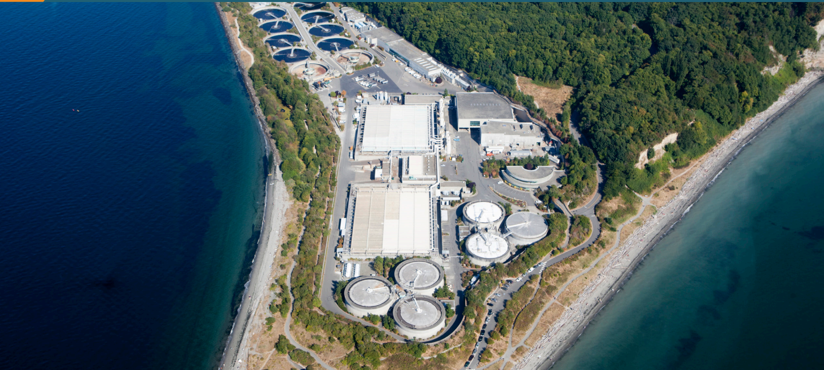
West Point Treatment Plant. Credit: Carterdayne
