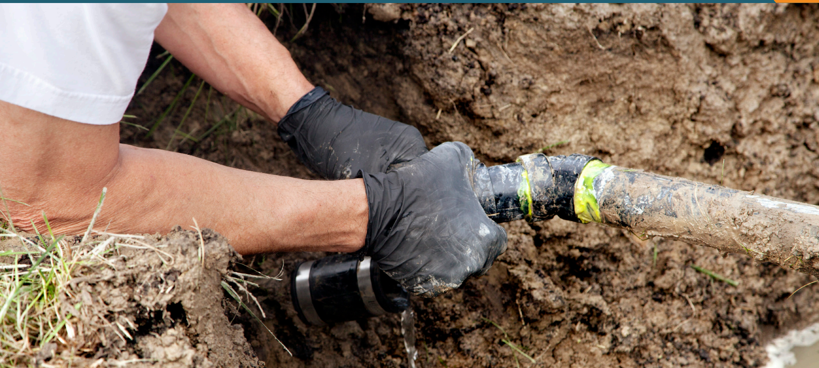
Repairing an onsite septic system. Credit: Lauripatterson
