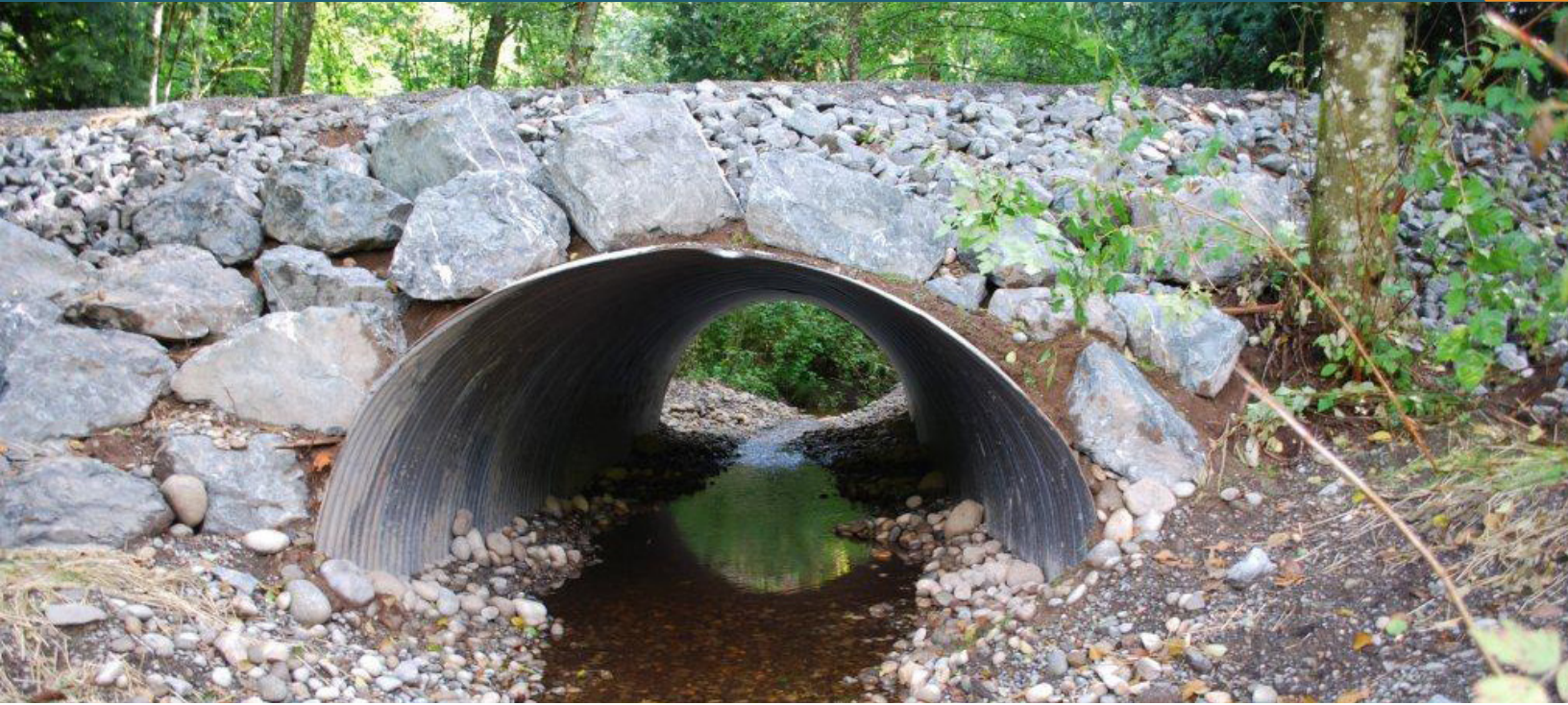
This new bridge allows trout, salmon, and other fish upstream access. Credit: Washington State Department of Natural Resources
