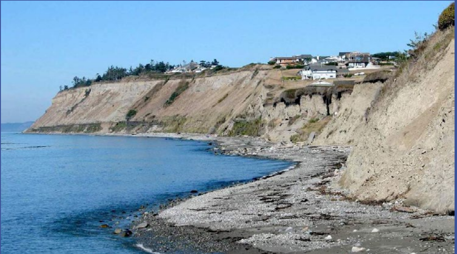
In addition to flooding, sea level rise can contribute to coast erosion as seen at the base of the bluffs north of Libbey Beach Park on the west side of Whidbey Island. Photo: Ecology (CC BY-NC-ND 2.0)
