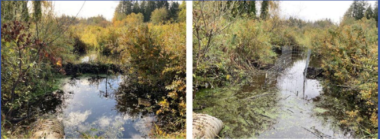
Caption: A beaver dam before and after notch exclusion fencing was installed to promote water flow and manage water levels on a tributary to Stevens Creek in Lake Stevens. Photo: Courtesy Snohomish Conservation District
