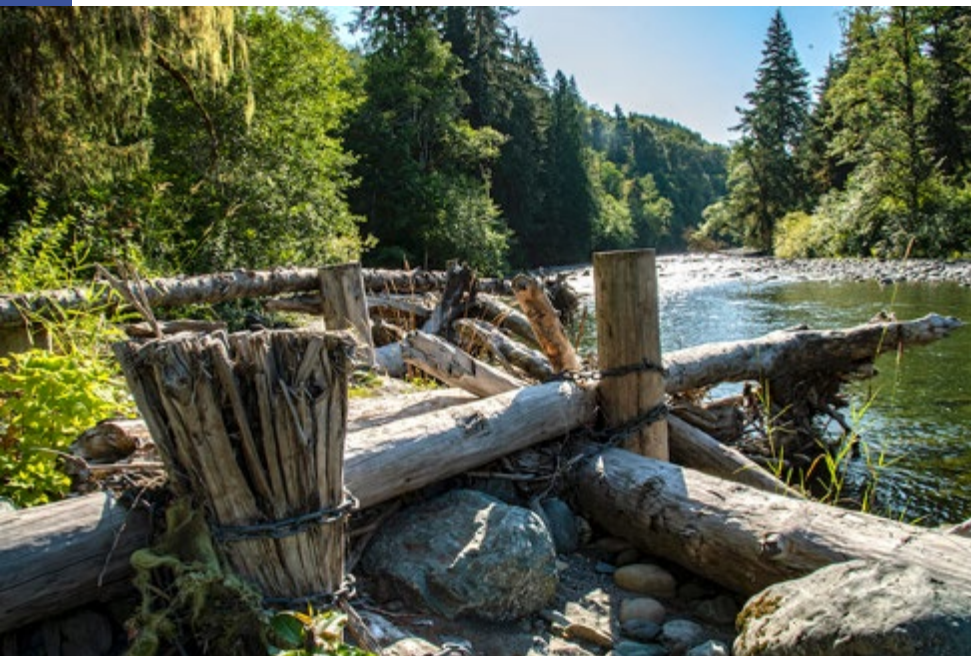
Engineered log jams like this one installed in the South Fork Nooksack River can reduce the risk of flooding by slowing down the flow of the river. Photo: Lance Cheung/USDA NRCS
