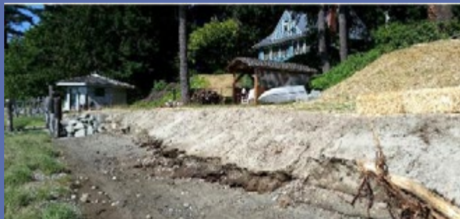
Property in Dyes Inlet before (top) and after (bottom) bulkhead removal (NTA 2018-0322).
