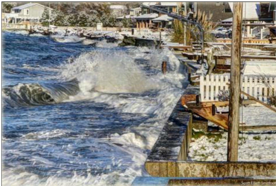
Storm surges against the bulkheads protecting beach houses at Mutiny Bay, WA. Photo: Scott Smithson (CC BY-NC-ND 2.0) https://www.flickr.com/photos/dtwpuck/15725058917
